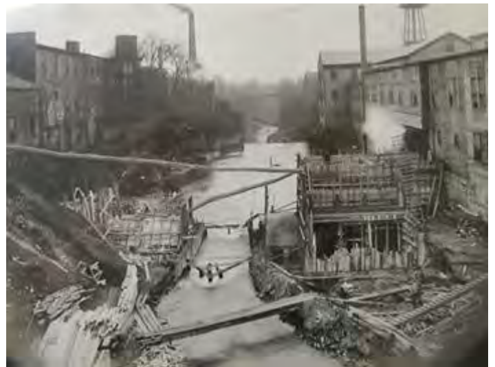
Construction photograph of Mill/Sheraton Dam, ca. 1914, looking south
