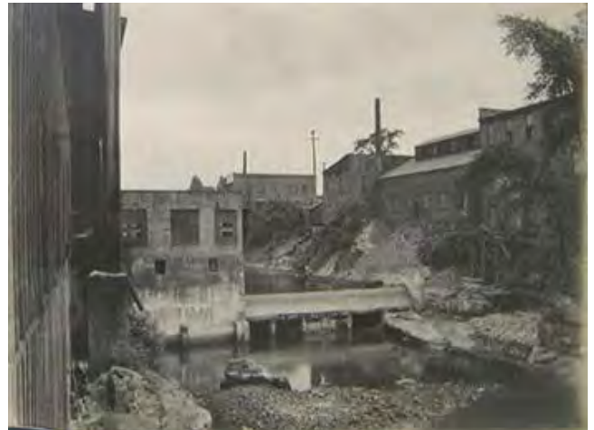
Completed Mill/Sheraton Dam, post 1918, looking north
