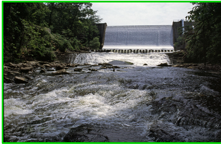
The Great Falls of the Cuyahoga River in Gorge Metro Park Dam built in 1914
