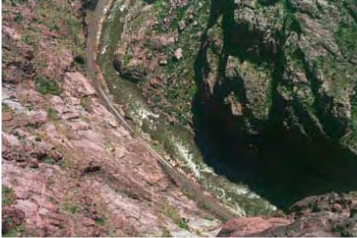
Below the Royal Gorge Suspension Bridge
