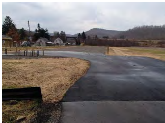
Entry driveway and improved area in the background. Note the new ditch down the middle of the field.
