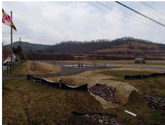
Drainage ditch along the east fence and paved access path to the liquor store.
